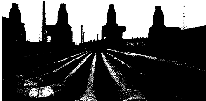
Figure 14: A pump station with four pumps (photo by Sergei Grits [144])
