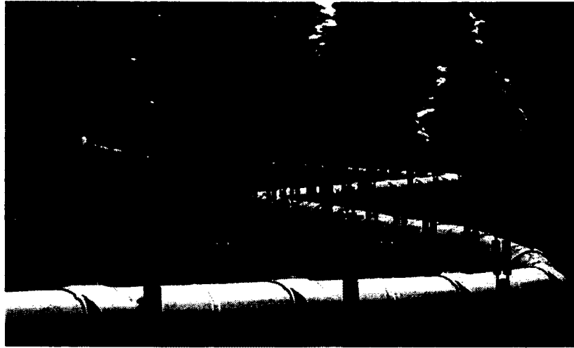
Figure 12: Snapshot taken from Alaska pipeline (taken from [141])
